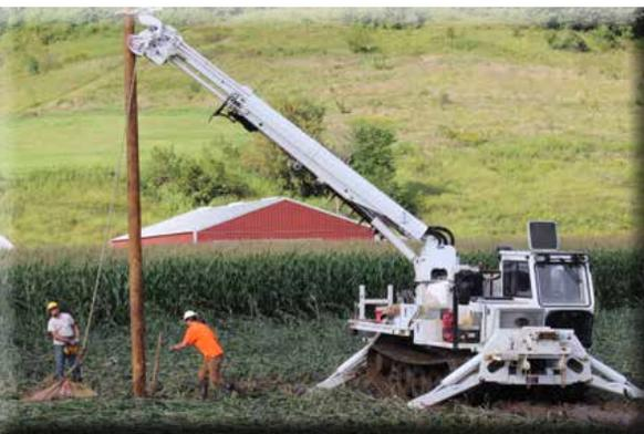
Track vehicles became indispensable to access flooded areas to make repairs. Vernon Electric has one track vehicle and borrowed three more from other co-ops.
