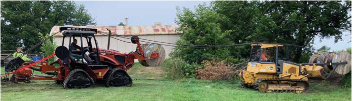
Above and right: If conditions and cost allow, some new line may be installed underground. VEC contracts with A-1 Power to assist with underground cable plowing. Here they are plowing new cable near a new solar array by Red Mound.
