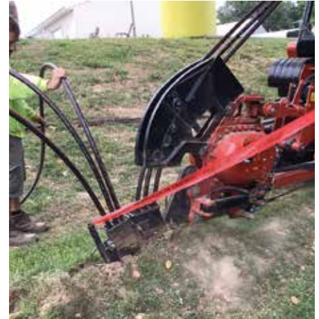
Above and right: If conditions and cost allow, some new line may be installed underground. VEC contracts with A-1 Power to assist with underground cable plowing. Here they are plowing new cable near a new solar array by Red Mound.
