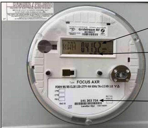
Your meter reading appears here. In this example the meter reading is 4152.
